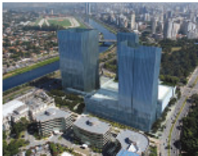
The JK complex in São Paulo will consist of Villa Daslu, a 250-store shopping center and three office towers.
